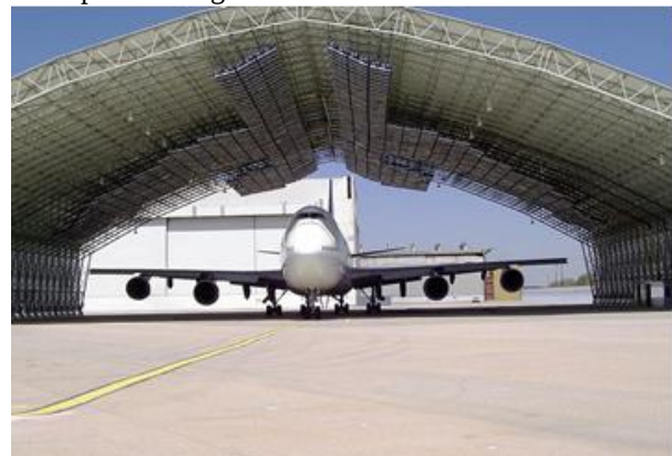
Fig. 8 Infrared hangar at New York JFK airport
